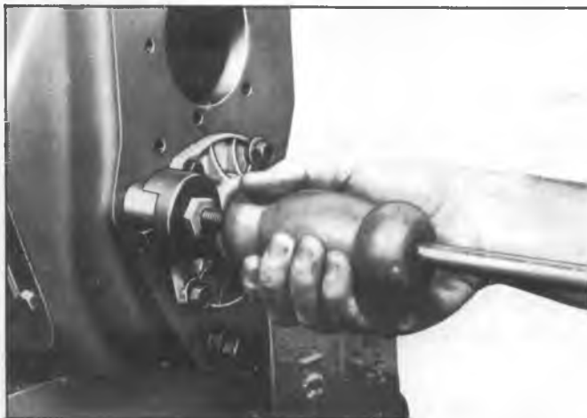
Fig. 3NP-Removing Reverse Idler Shaft
